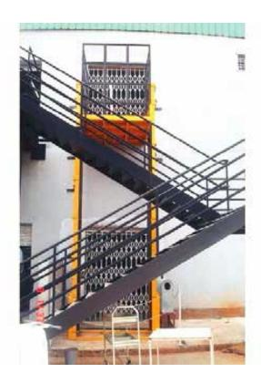
Joist dual mast hydraulic goods lift is widely used to transfer material from one floor to another. It is to be installed with wall support at the one side and rest 2 sides can be used for loading & unloading purpose.
